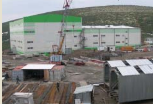
Construction of main building
